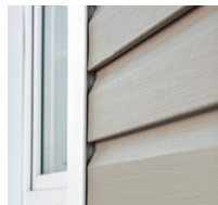
Siding, Window & Door Installation
