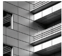
Metal Roofing & Wall Panel Installation
