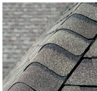
Residential & Commercial Roofing
